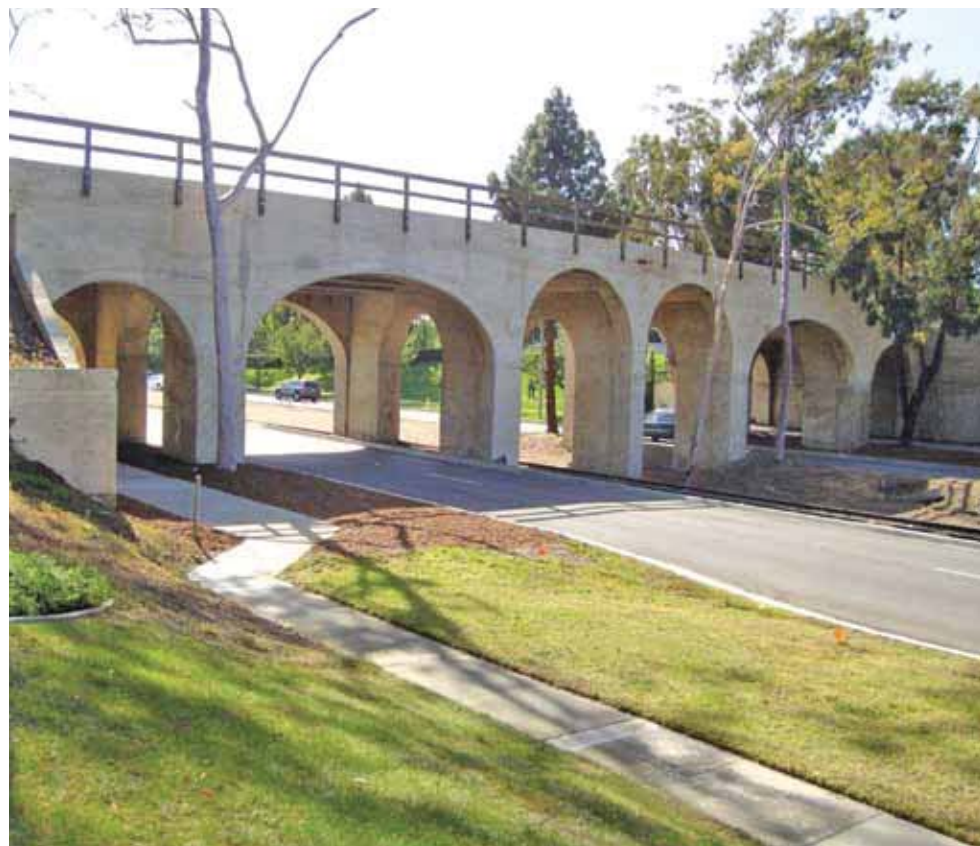
The now dedicated Pacific Electric Railway El Prado Bridge.
